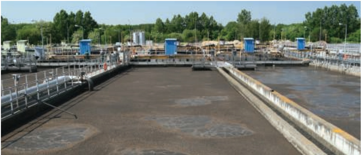
FIGURE 2. Wastewater treatment often involves settling of solids in a tank such as this one
