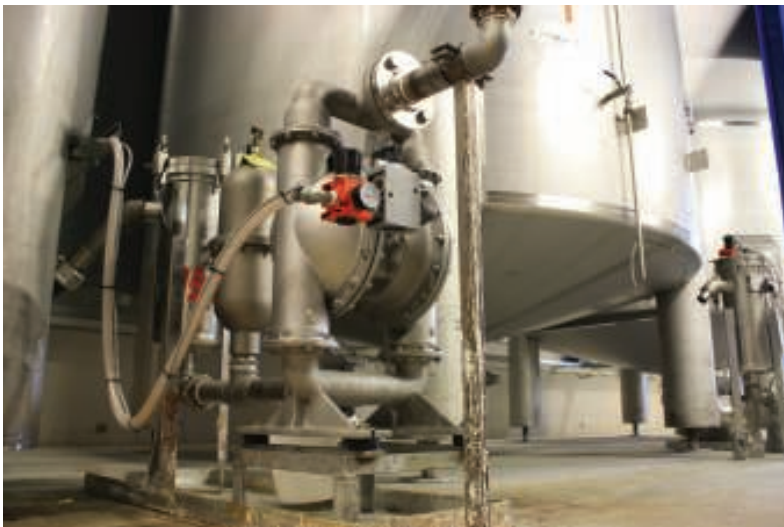
FIGURE 6. A major advantage of AODD pumps is the simplicity of their integration into existing plant footprints
