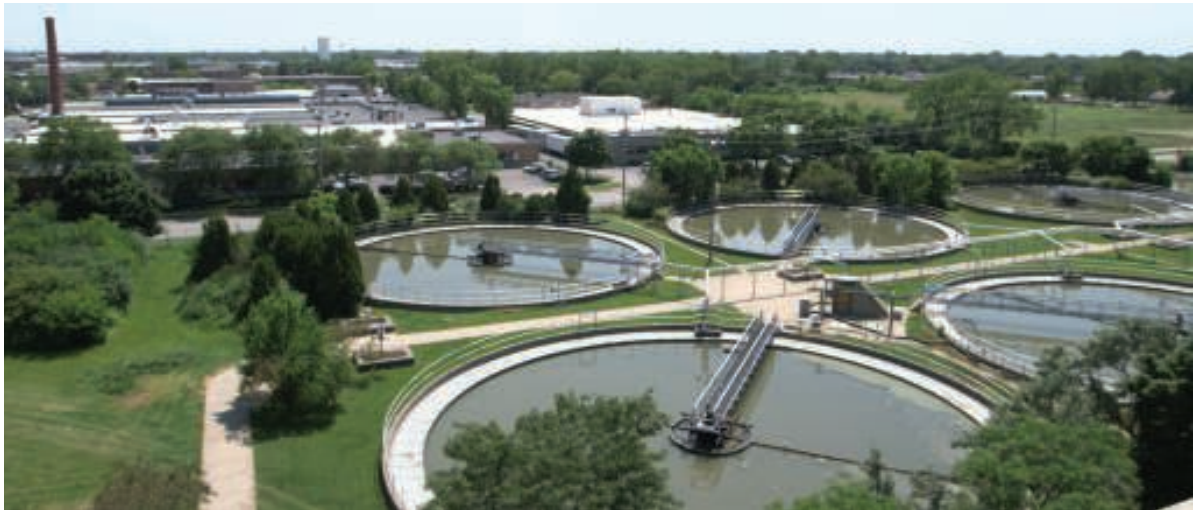
FIGURE 3. The flocculation and coagulation steps, which allow small microbial flocs to form and join together for removal by clarification is achieved through a combination of chemical addition and physical separation
