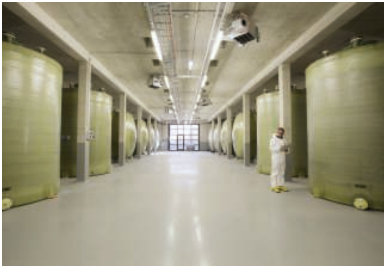
FIGURE 2. Shown here is the installation of the storage tanks that will hold acidic vanadium solutions for the 3-MW RedoxWind project in Pfinztal, Germany
