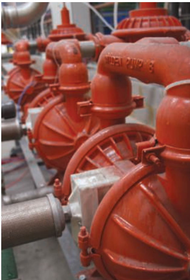
FIGURE 1. AODD pumps can handle a wide variety of materials, including very viscous media, and can also pass large solids
