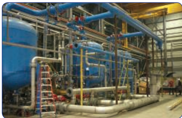
An Ovivo boiler-water treatment plant under construction
