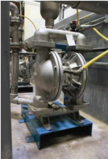
FIGURE 5. AODD pumps' flow paths can be optimized to further reduce air consumption
